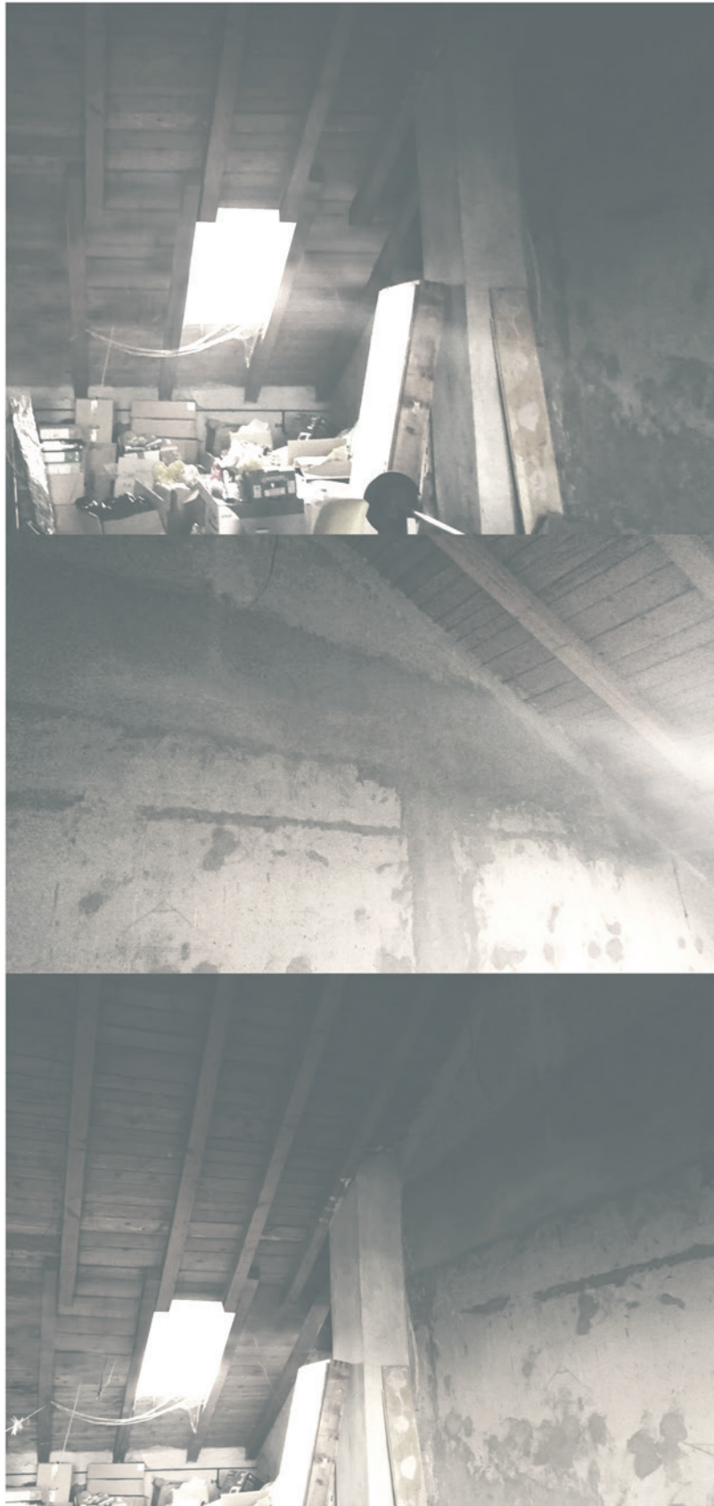
dark space before renovation
